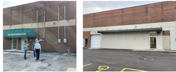
A much needed overhaul of the parking lot has been completed.
